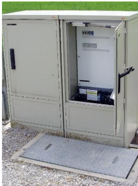
Figure 7: coffret autoportant en aluminium (Exemple)
